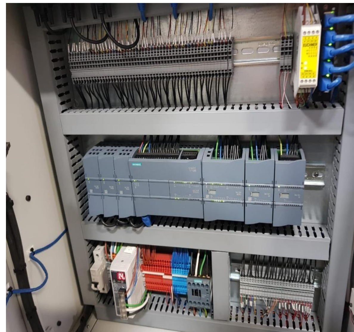
Control cabinet, PLC, regulators, terminals, input and output labeling.
